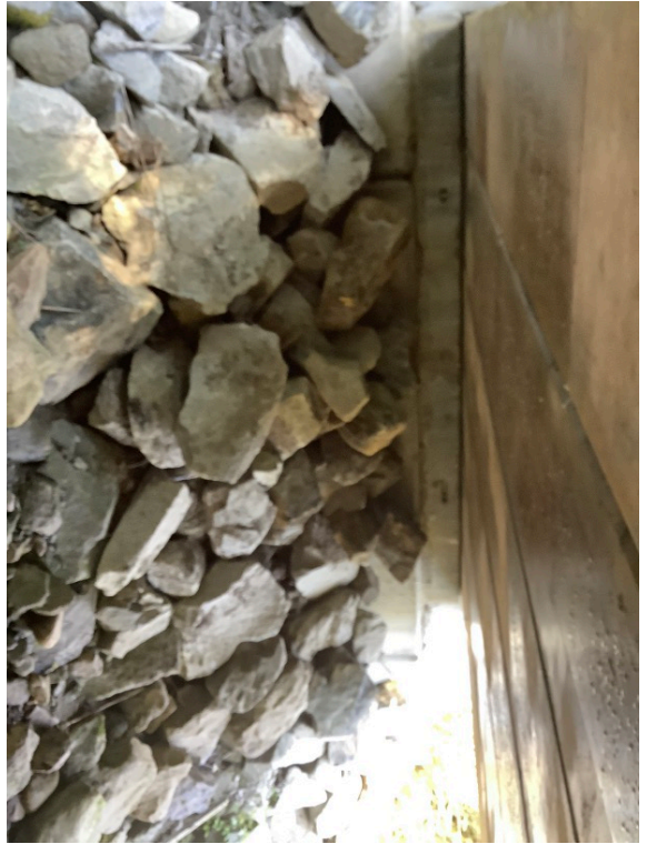
Left Bank Abutment when facing downstream
