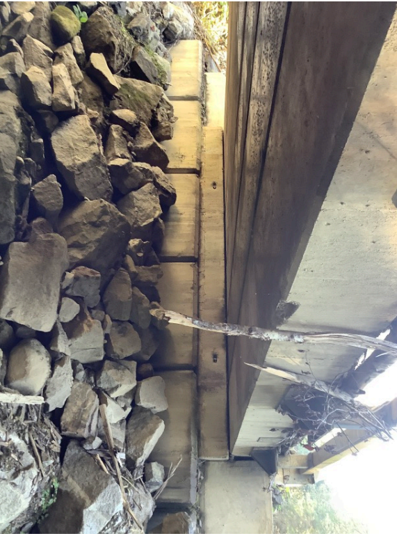
Right Bank Abutment when facing downstream
